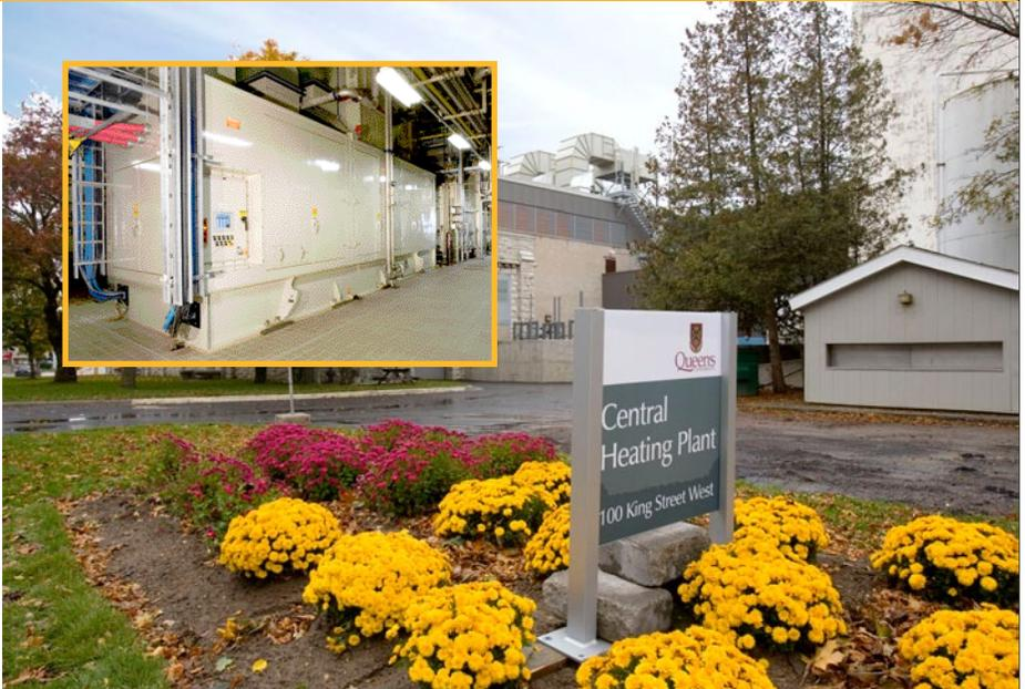
The predominant heating and cooling design favored by universities worldwide is the “district” approach, in which multiple buildings are supplied chilled water and heat from a central plant. Cogeneration systems are capable of providing not only heating and cooling, but power as well. And capitalizing on the benefits of cogeneration, the new plant will be more efficient than the combination of the older plant and the local electrical utility.
