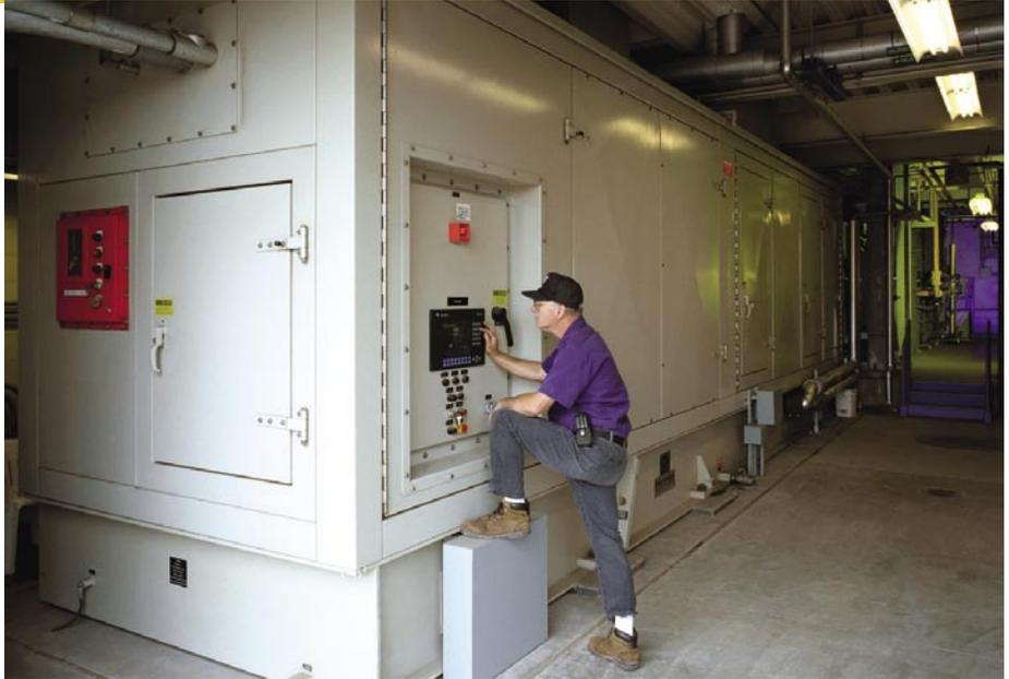
Seeking to manage its energy costs in a deregulated electricity market, while at the same time ensuring ultra-reliable, high-quality power to keep pace with its continuing growth, San Diego State University (SDSU) added an 11-MW cogeneration facility to its existing central plant complex.
