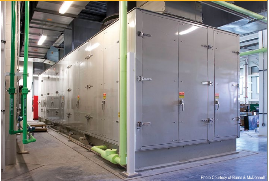
Photo Courtesy of Burns & McDonnell
